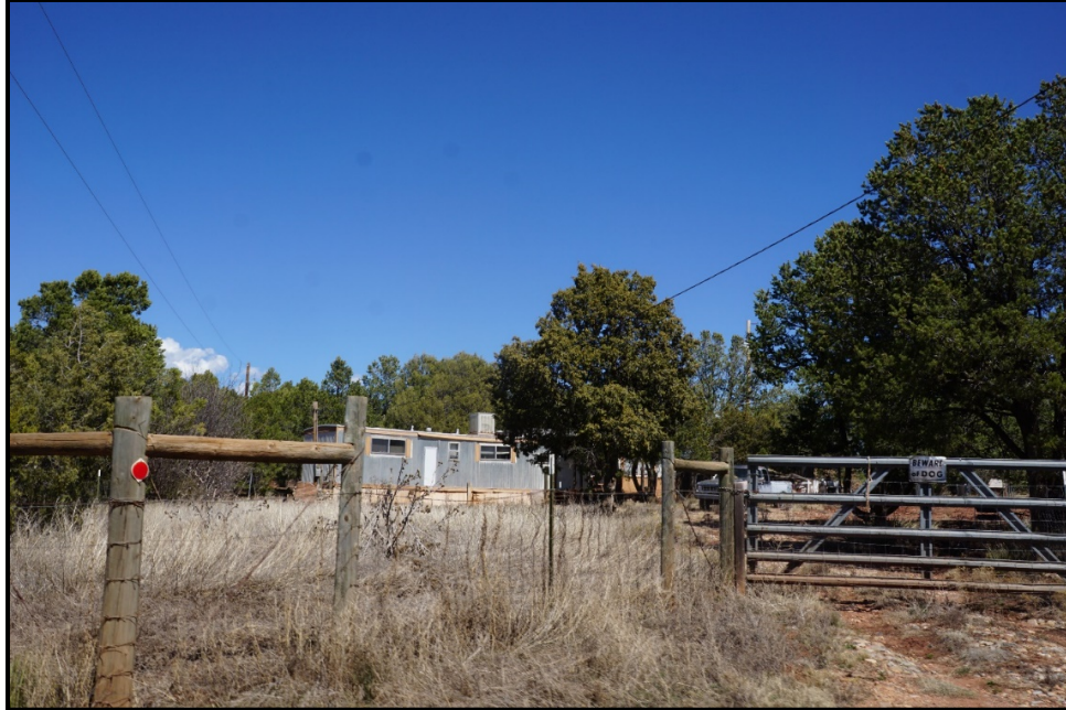
Figure D.29. Poor defensible space within the La Jolla area.
